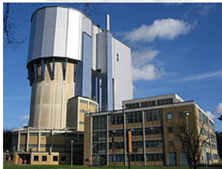
Image 1: Reactor building with material gat
