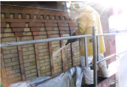
Image 4: Trainees cleaning with the torbo system We agreed to support this project with two of our machines. They started in the beginning of October.
